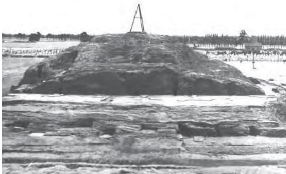
Fig. 1. Lingtai Central Platform Foundation Site
