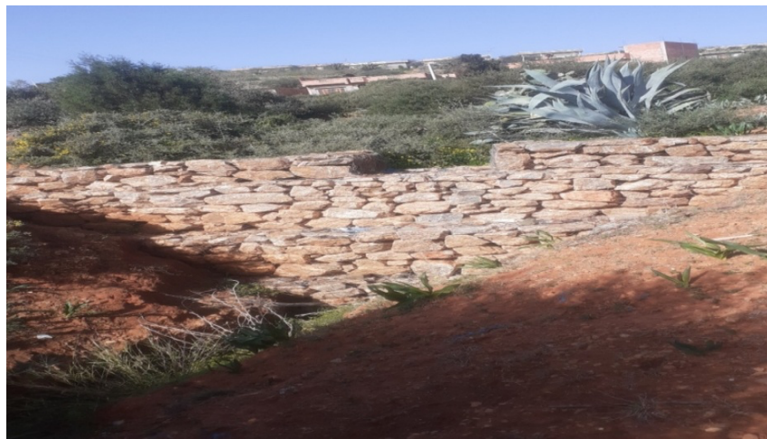
Photo 13: Stable gabion threshold with two cages and a rectangular spillway in the Ain Merika station
