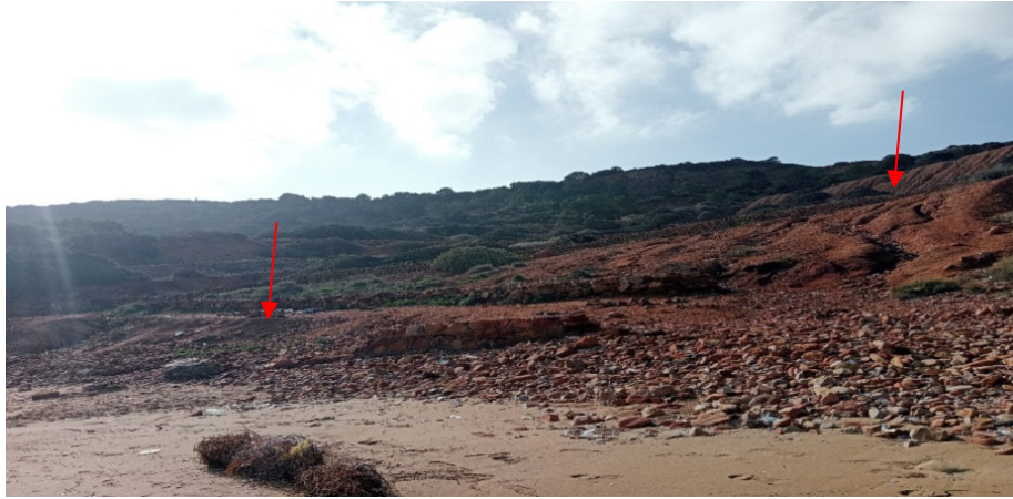
Photo 12: Acceleration of the erosion phenomenon following the instability of gabion sills
