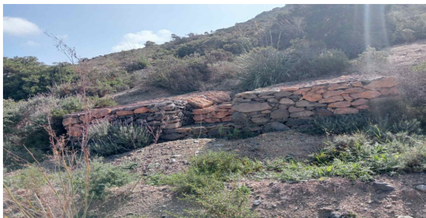
Photo 14: Stable gabion threshold in the Ouled Ben Ayed station
