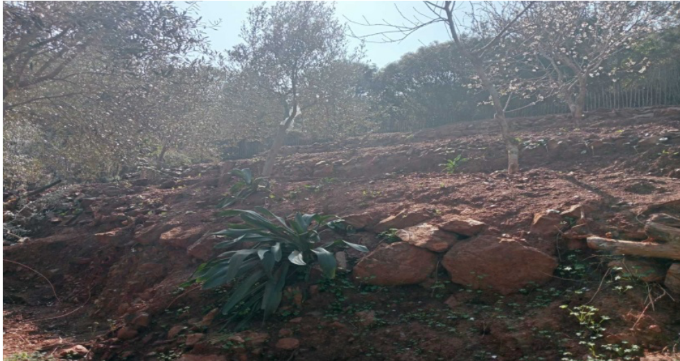
Photo 15: Low walls built in station 5
