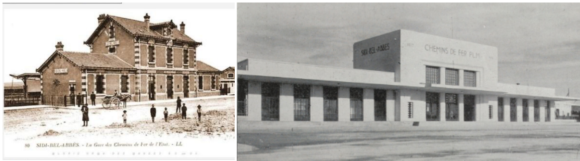
Fig. 8. Old and new Sidi-Bel-Abbès railway station (Archive of Railway Transport)
