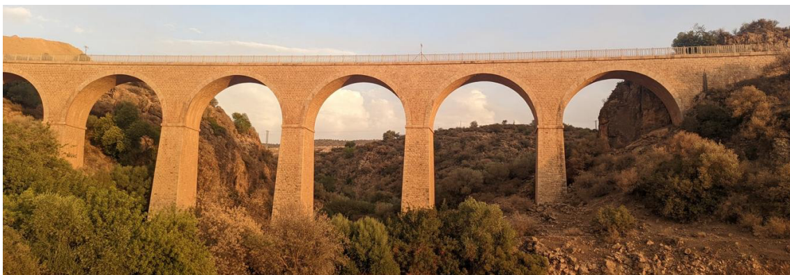
Fig. 14. masonry viaduct with six 15 m arches over the Oued Ksab (Dahmani. M, 2023). (Archive [SNTF])
