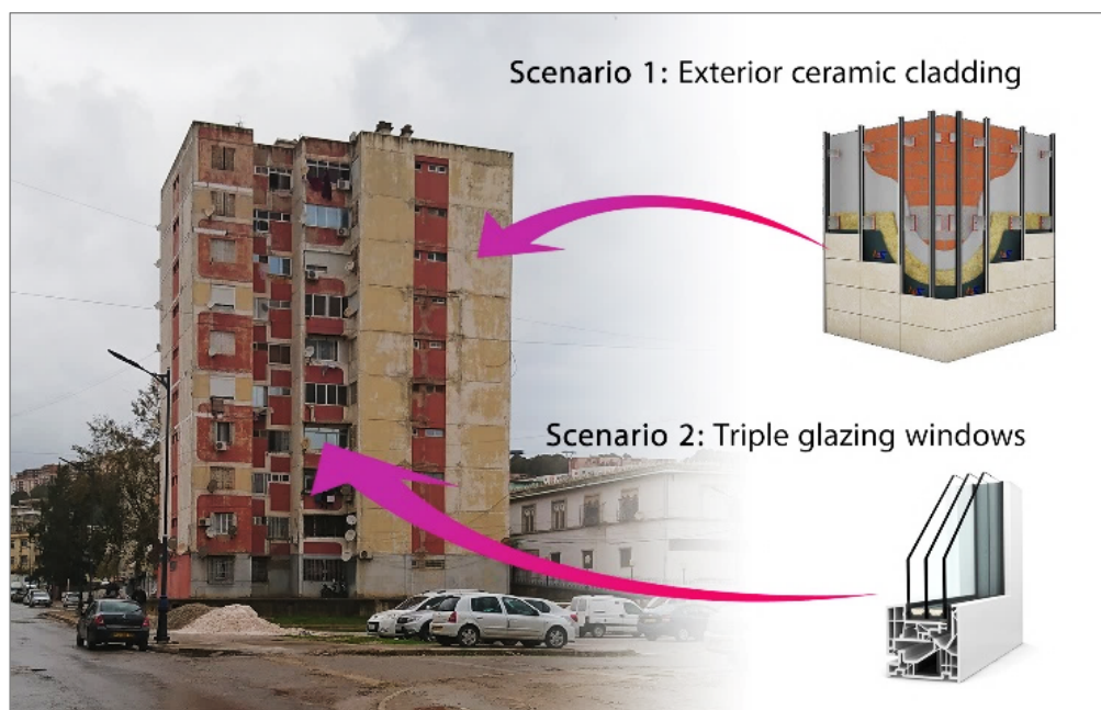
Fig. 3. Photographic shot of the case study, with the two scenarios for intervention on the building's external envelope.
