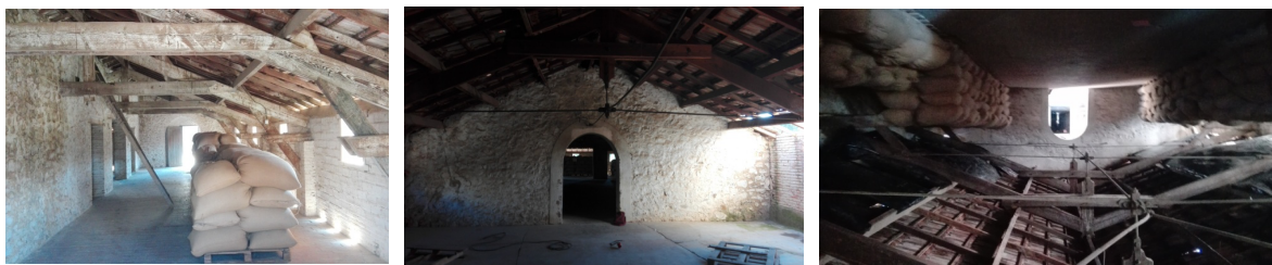
Figure 5. A well-preserved state inside the warehouses with the wooden framework in good condition. (Source: author).
