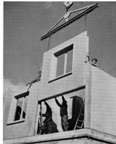
Figure 4. Samiex approved by the CSTB in 1956, Orleans site (CNAM, 2009), (d) Overview of a floor under assembly and an example of the assembly of a standardized facade element (Nogue, 2014).
