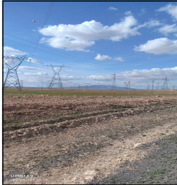
Photo N 0 04: High-voltage power lines are widely distributed in the western and southern parts of the city.
