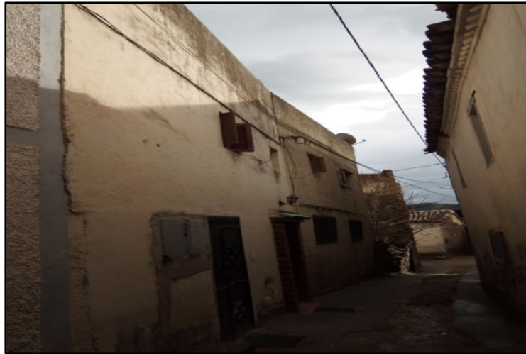
Figure 11. Façade of the house Case N°04 (authors).
