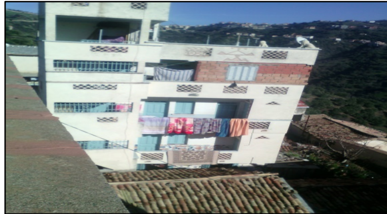
Figure 8. A building showing case N°03 (authors).
