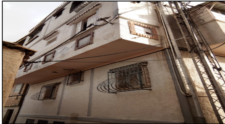
Figure 10. Façade of a house Case N°04 (authors).
