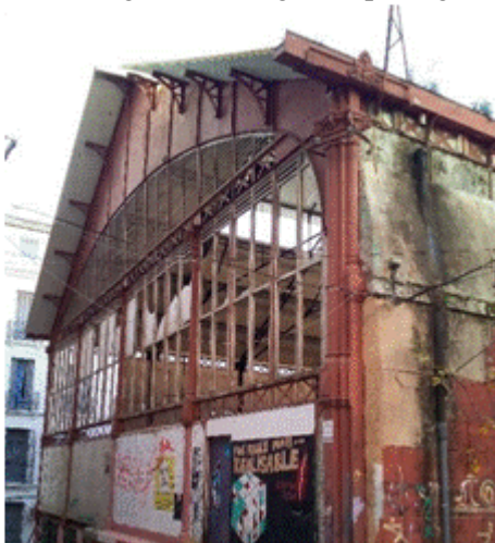
Figure 5. "Halle Volta", East Façade. Source: authors, 2022.
