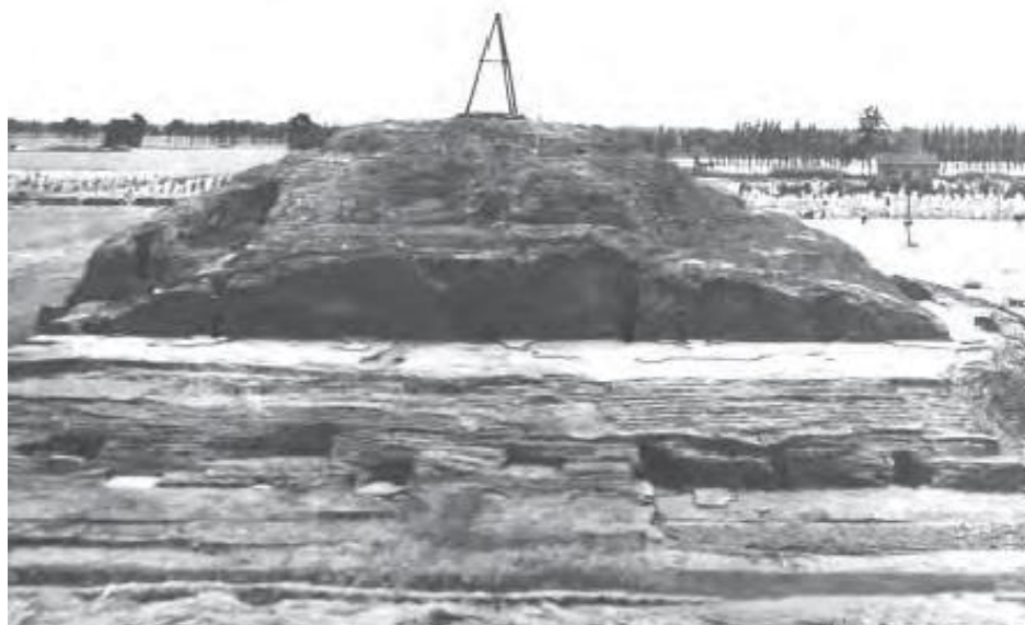
Fig. 1. Lingtai Central Platform Foundation Site
