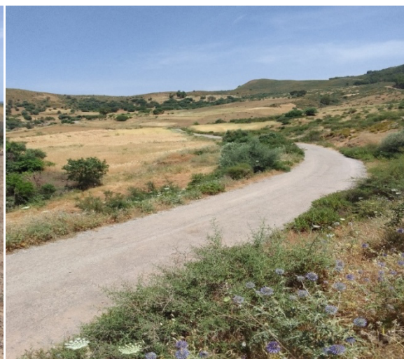
Photo 2. Track opening with surfacing
